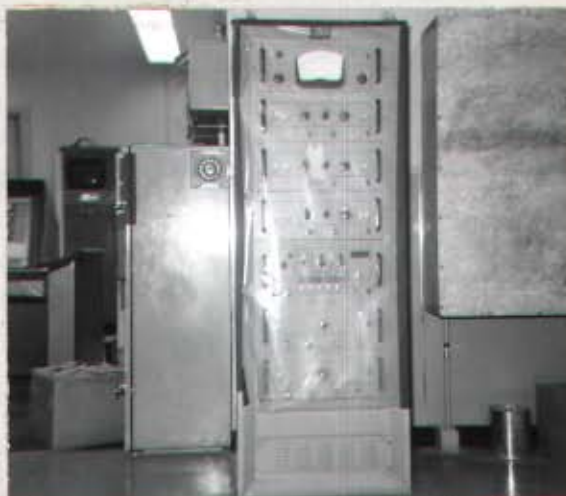
Site 4, Cortland. BDS Console in position to be hooked up is protected from dust and moisture by Polyethylene cover.
