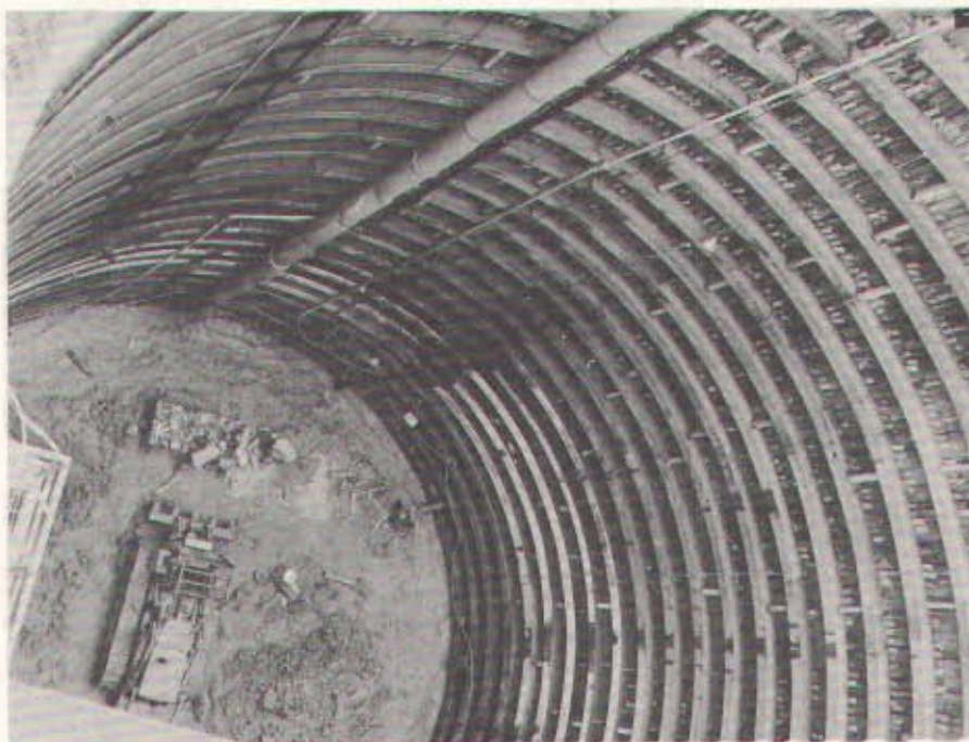
Site 1. Interior view of missile silo. Depth of silo excavation is 85 feet.
