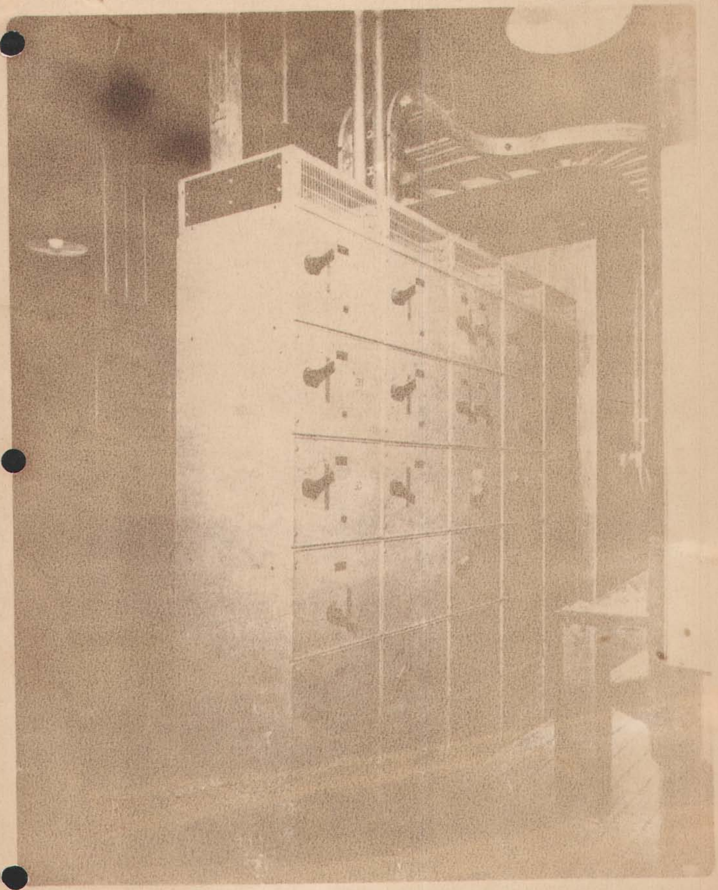
Figure 2 Non-essential Motor Control Center - Rear View
