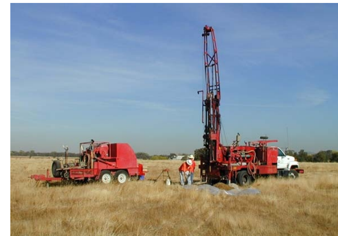
Drilling contractors collecting soil and groundwater samples during the Church property investigation
