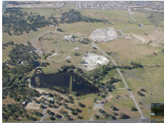
Aerial view of the Titan I-A Missile Facility
