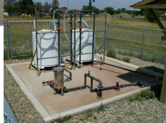
Titan I-A groundwater treatment system
